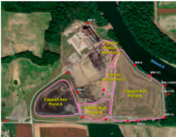
HUTSONVILLE COAL ASH PONDS
