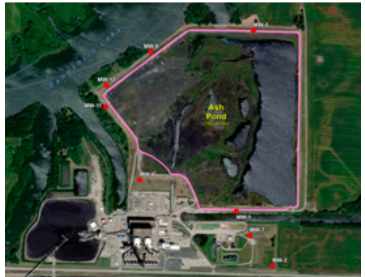
KINCAID COAL ASH POND
