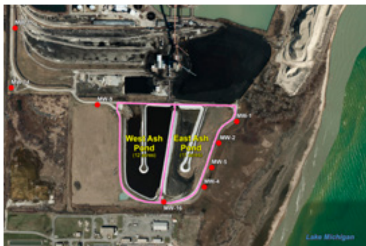
WAUKEGAN COAL ASH PONDS
