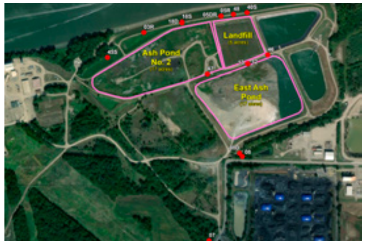
HENNEPIN EAST COAL ASH PONDS
