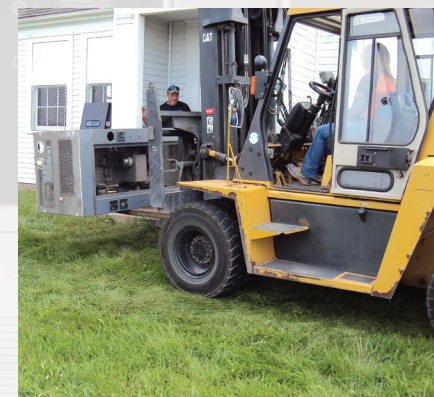
Old WILL-AM transmitter being removed
